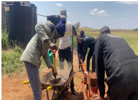
Bricks Making at Huri Hills
